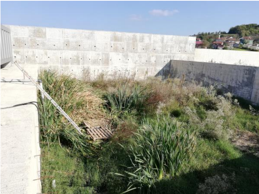
Kutlubey Campus Package Treatment System
