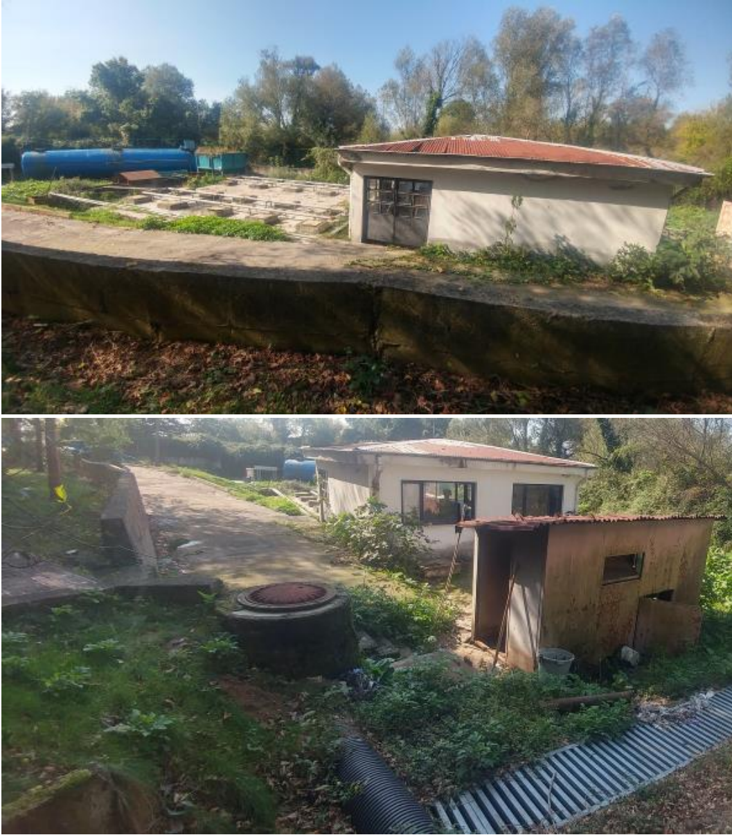
Ağdacı Campus Treatment Plant
