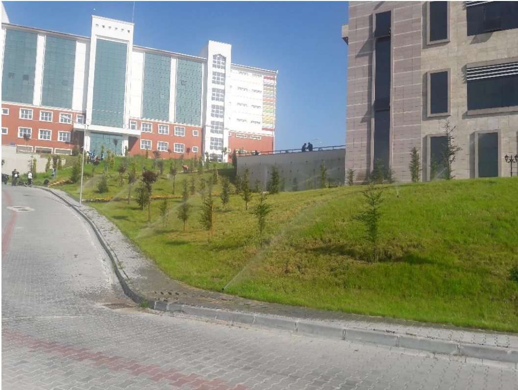
Automatic irrigation systems
