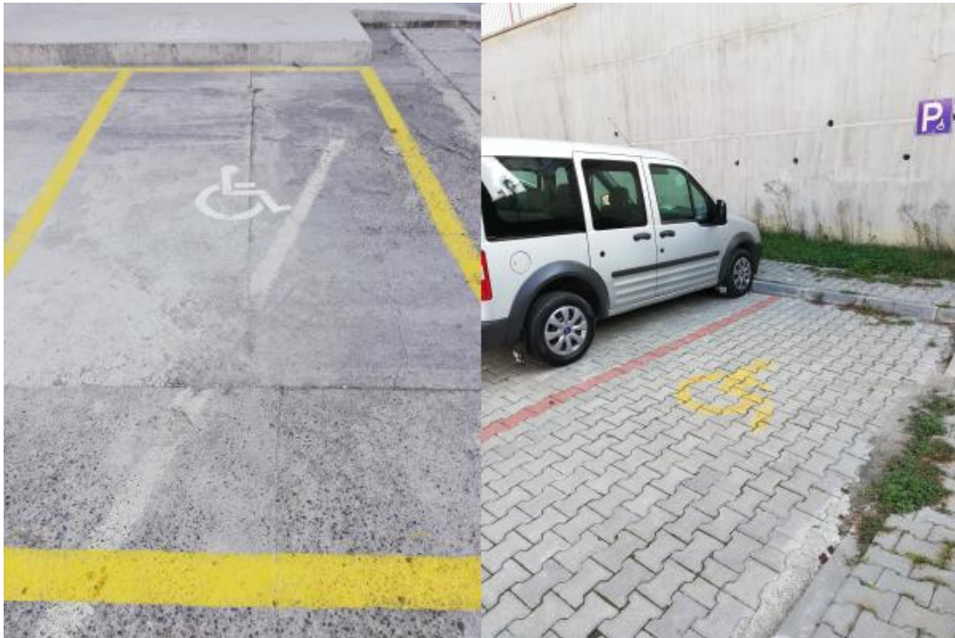
Sidewalk, road and building entrances on campuses are designed to be disabled and pedestrian friendly
