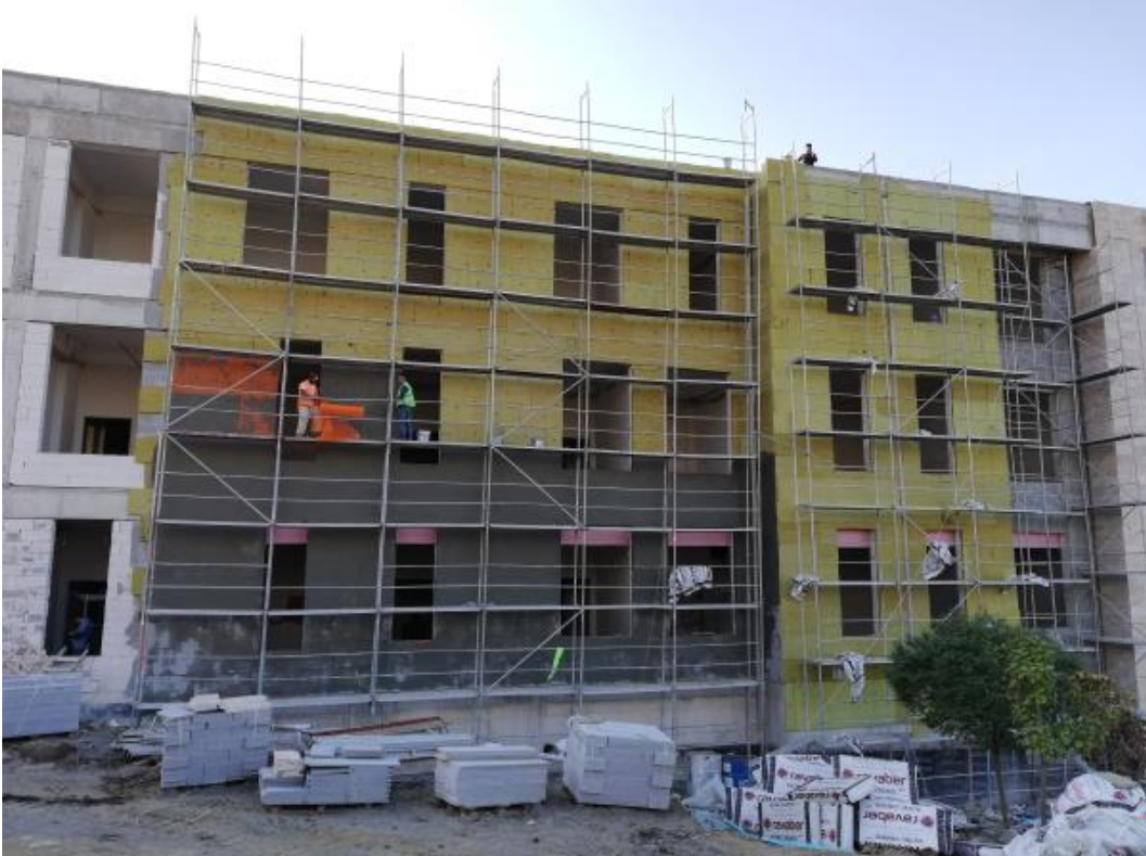
The newly built buildings on the Kutlubey Campus are insulated
