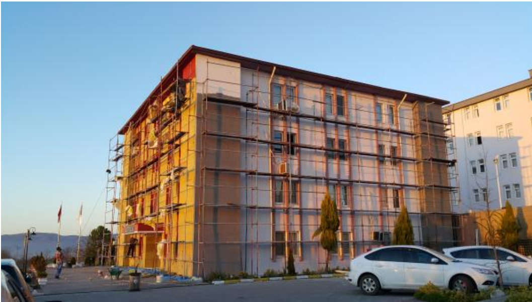
The old buildings in Ağdacı Campus.were made energy efficient by making insulation
